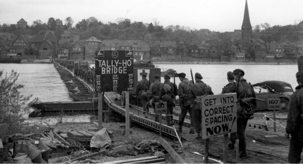
Left: The 6th Airborne Division crossing the River Elbe on April 30th, 1945 into the town of Lauenburg. Notice the large vehicles and careful spacing on this long pontoon bridge.
